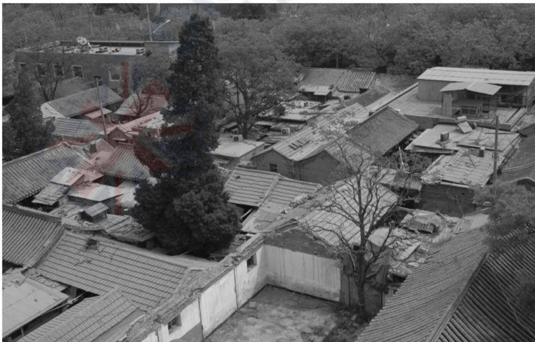
Fig. 11- 3 Informal constructions filling in traditional courtyards
