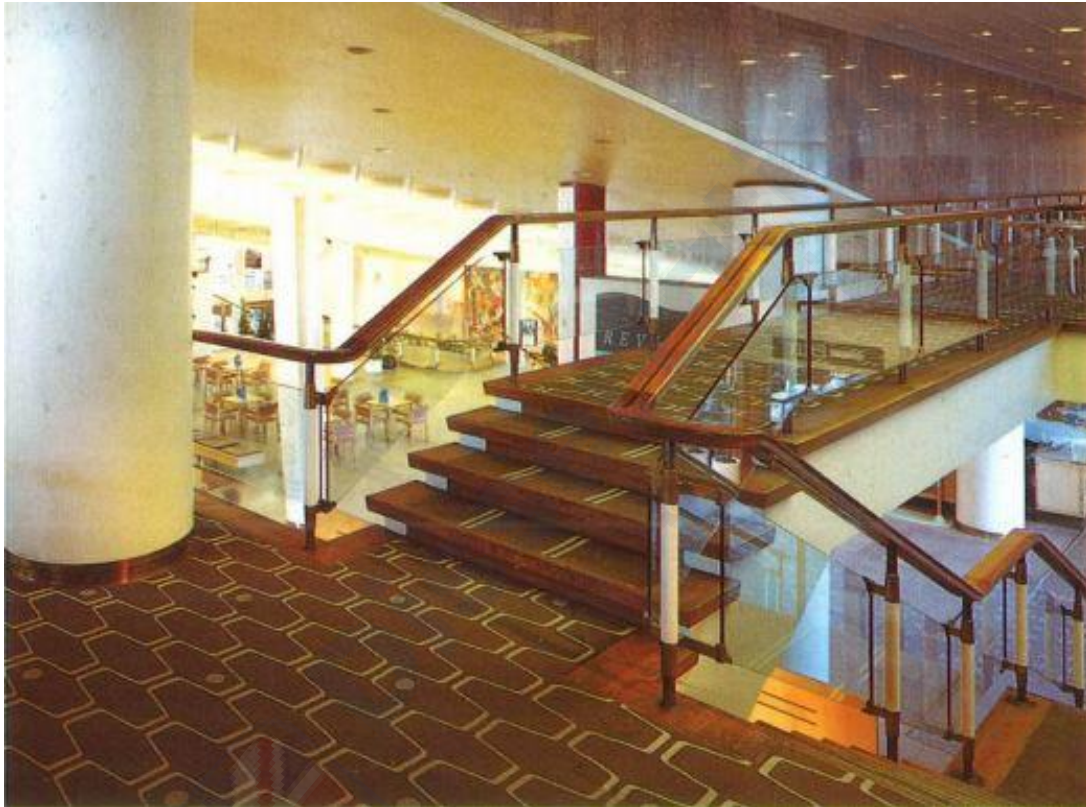
Fig. 7- 8 The foyer spaces after the refurbishment
