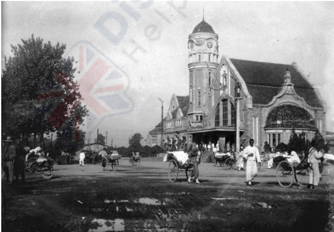
Fig. 5- 3 Jinan Station for Jin-Pu Railway, 1930s
