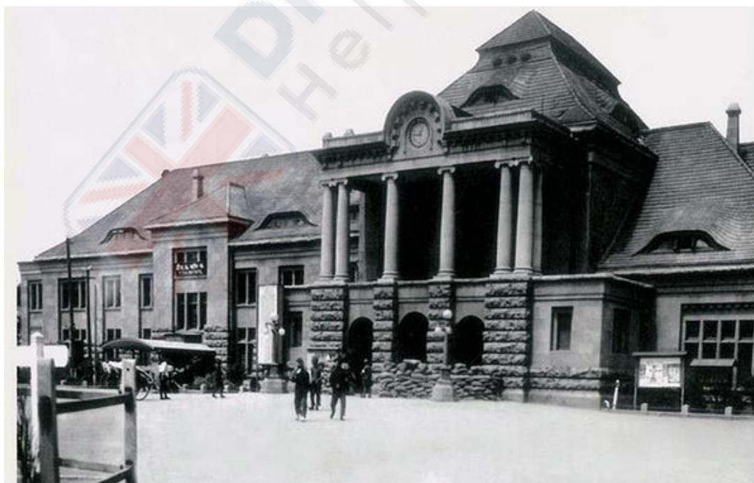
Fig. 5- 5 Jinan Station for Jiao-Ji Railway
