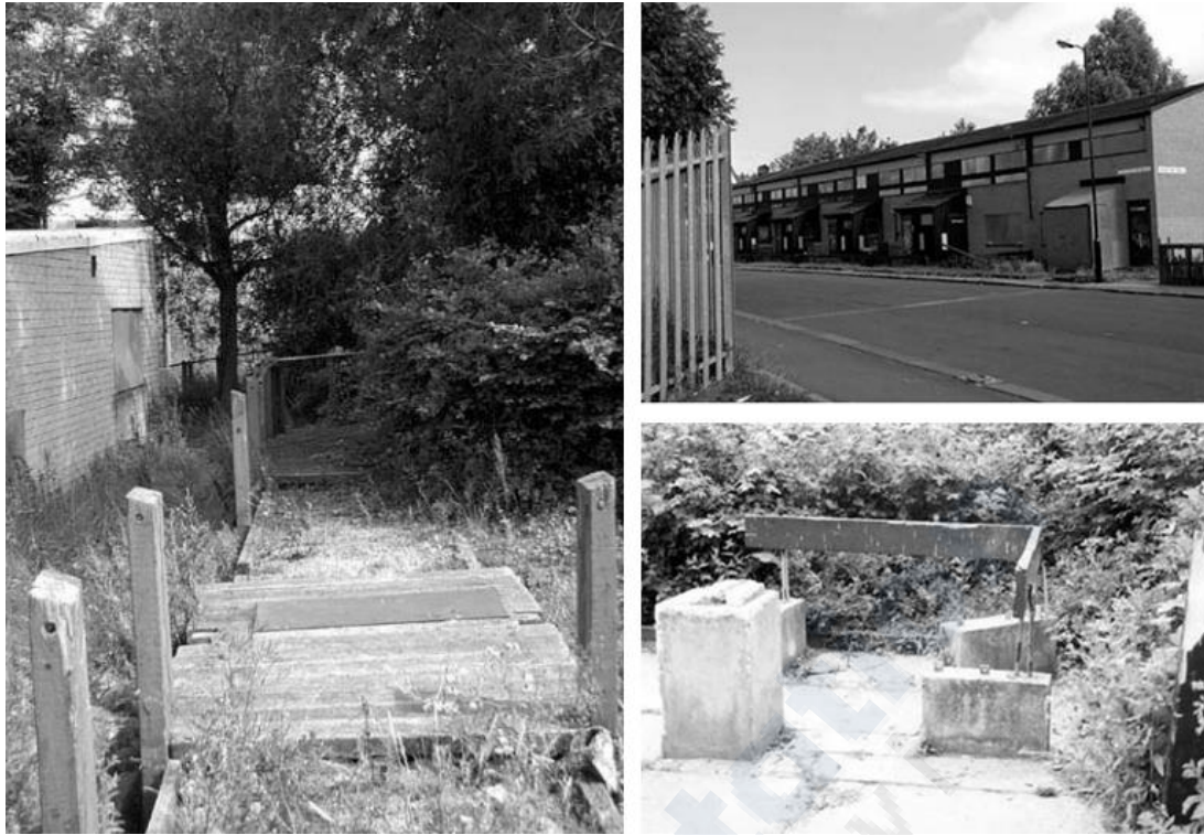
Fig. 10- 4 Dilapidated housing and environment, around 2001
