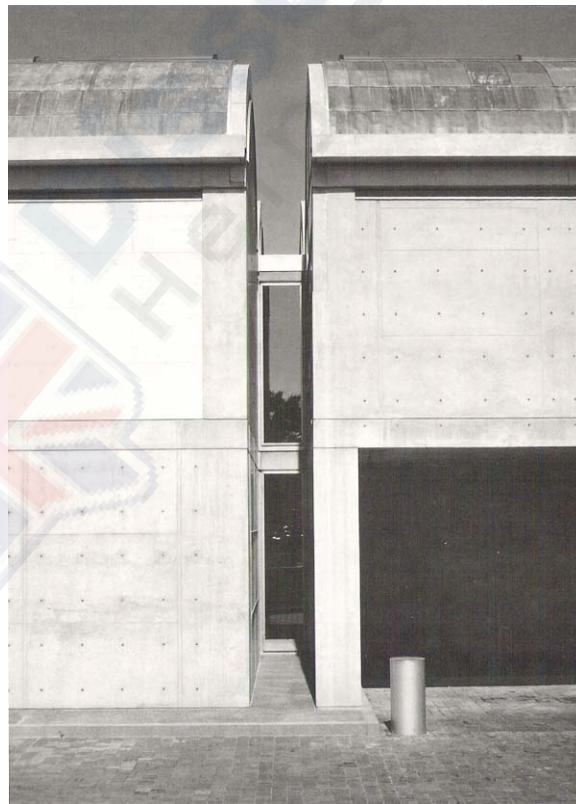
Figure 4.21: A Kimbell glazing interval. It is the tectonic of junction. (Source: Nell Johnson, Light is the Theme, Louis I. Kahn and the Kimbell Art Museum , [Fort Worth: Kimbell Art Foundation, 2002], p. 42.)
